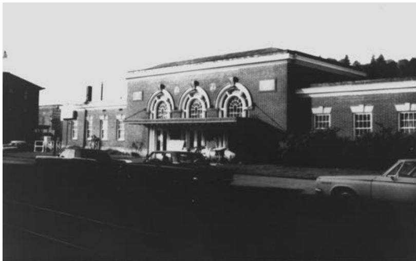
SWOMSI in downtown Eugene, OR in the old Oregon Electric Railway Station located on the corner of Willamette St and 5 th Avenue.
